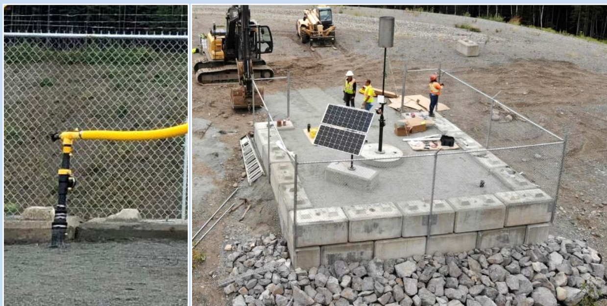
Photos 1&2 - QED Precision Wellhead (left) and Solar Spark Flare at the Thornhill Landfill (right)
