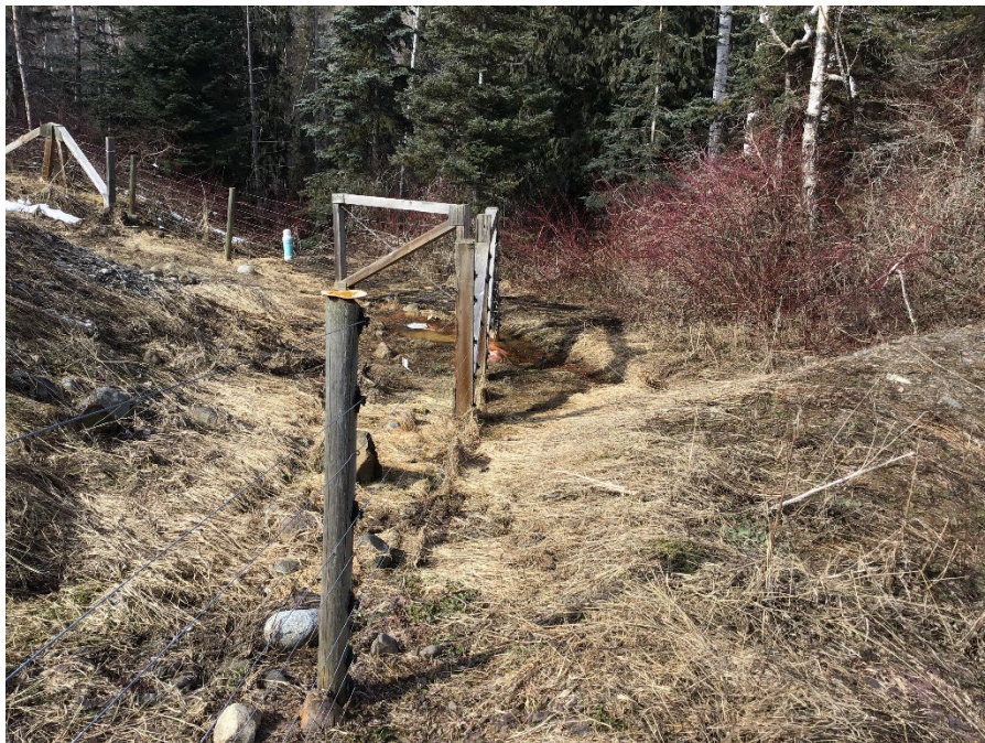
Photo 6: Kitwanga Landfill leachate breakout near northwest corner of landfill, looking west, April 13, 2022
