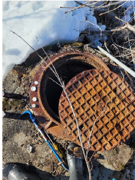
Photo 9: Meziadin Landfill SW-03, looking at manhole, April 12, 2022
