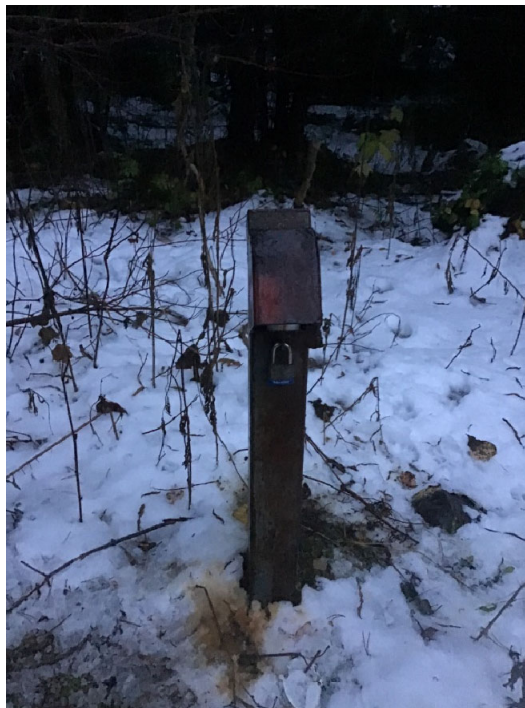
Photo 18: Meziadin Landfill MW-03, well monument, October 26, 2022
