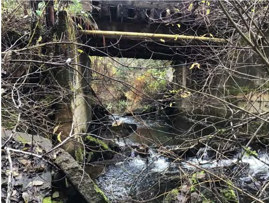
Photo 11: Thornhill Landfill SW-06, looking upstream, October 21, 2022
