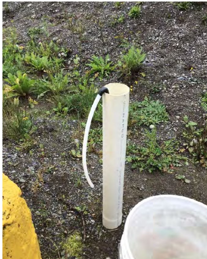
Photo 16: Thornhill Landfill MW21-01, October 20, 2022
